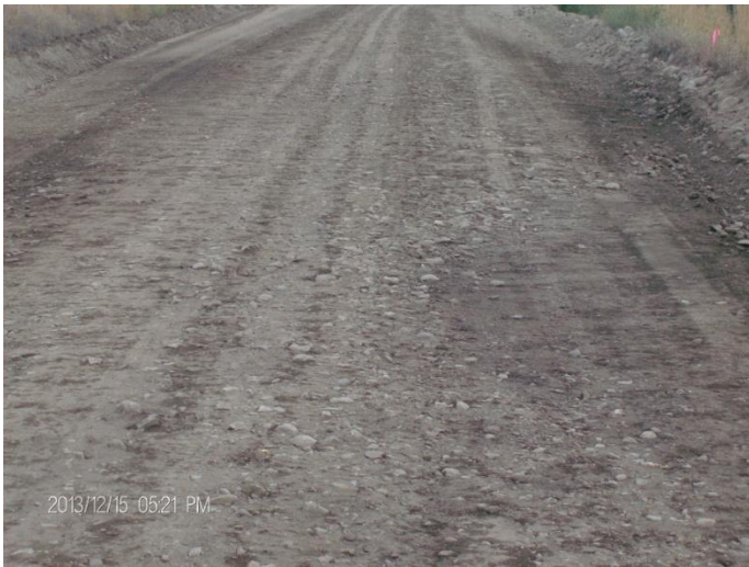
CUSTOMS RD.—PHASE TWO: IN PLACE LINEAR CRUSHING, Roadtech, Inc.
