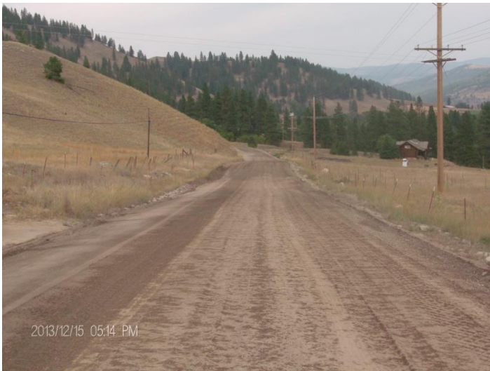
Phase Two, after final pull and process of ditch material. (Below)
