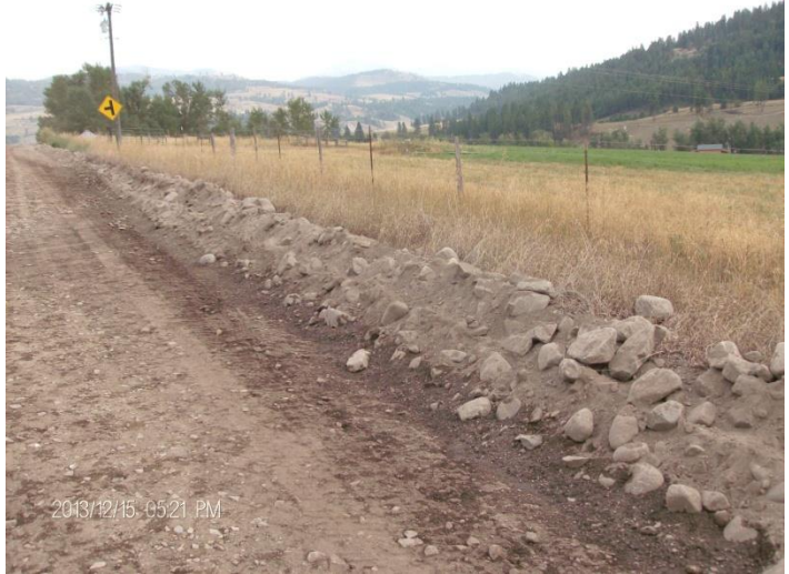
CUSTOMS RD.—PHASE TWO: IN PLACE LINEAR CRUSHING, Roadtech, Inc.
