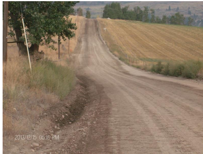
Phase Two, after final pull and process of ditch material. (Below)
