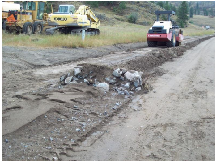
Oversize material from phase one staged in ditch to crush during phase 2. (Below left) (Below right) Typical road material 2 inch (-) after phase one.
