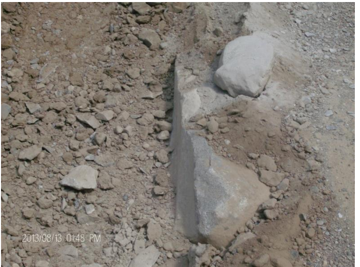
2 nd Pass, top 6" rock turned to gravel. (Below)
