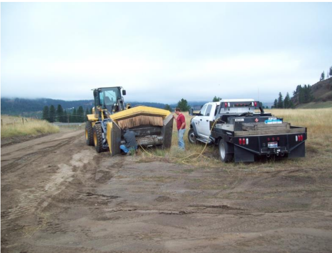
Oversize material from phase one staged in ditch to crush during phase 2. (Below left) (Below right) Typical road material 2 inch (-) after phase one.
