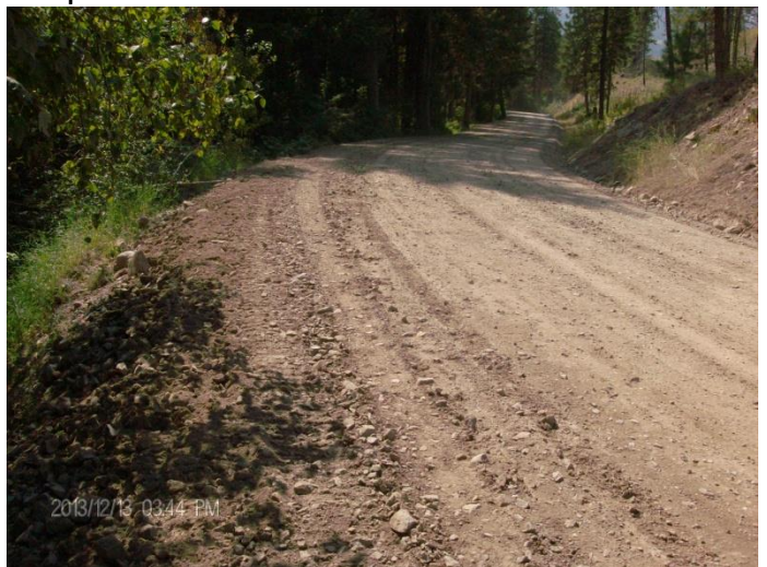
Oversize material from phase one staged in ditch to crush during phase 2. (Below left) (Below right) Typical road material 2 inch (-) after phase one.
