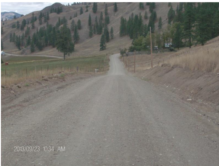
Phase Two, after final pull and process of ditch material. (Below)
