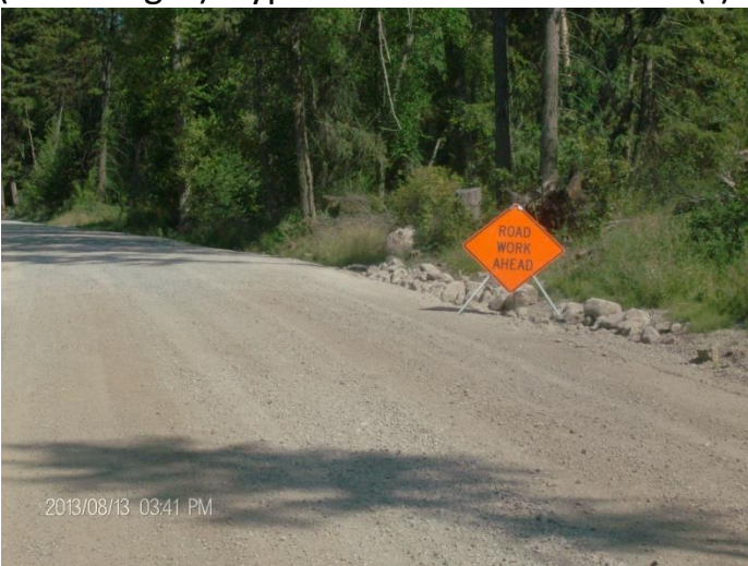
Oversize material from phase one staged in ditch to crush during phase 2. (Below left) (Below right) Typical road material 2 inch (-) after phase one.
