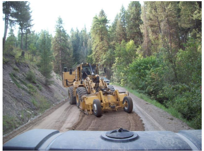
1 st Pass, rocks pulverized down 6". (Below)
