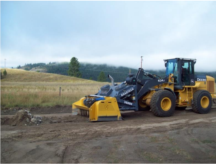
Crushing and shaping during phase 2. (Below)
